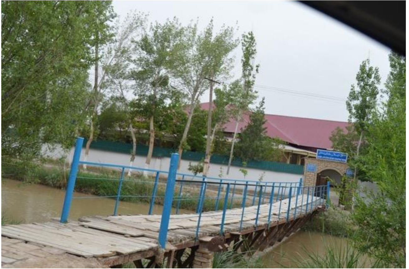
Picture 6: Pedestrian bridge at PK 262+00 (photo dated 04.03.2023)
