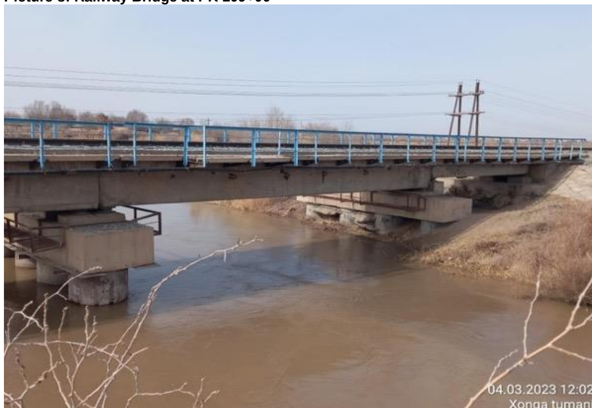
Picture 8: Railway Bridge at PK 109+00
