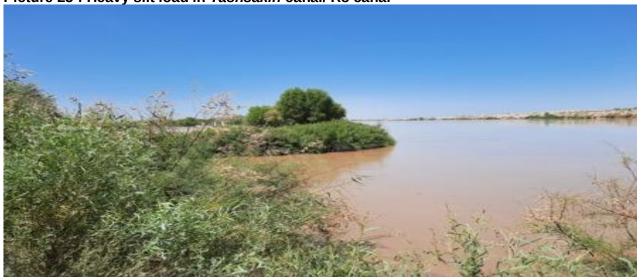
Picture 23 : Heavy silt load in Tashsakin canal/ R8 canal
