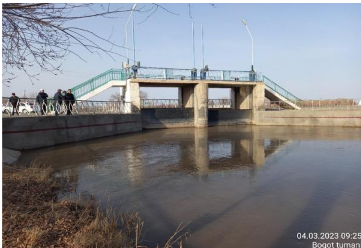
Picture 4: Head structure (PK 0+00)
