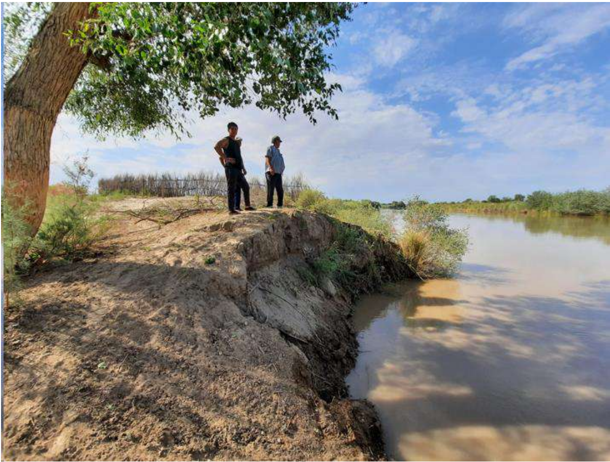
Picture 3: View of Bank Erosion
