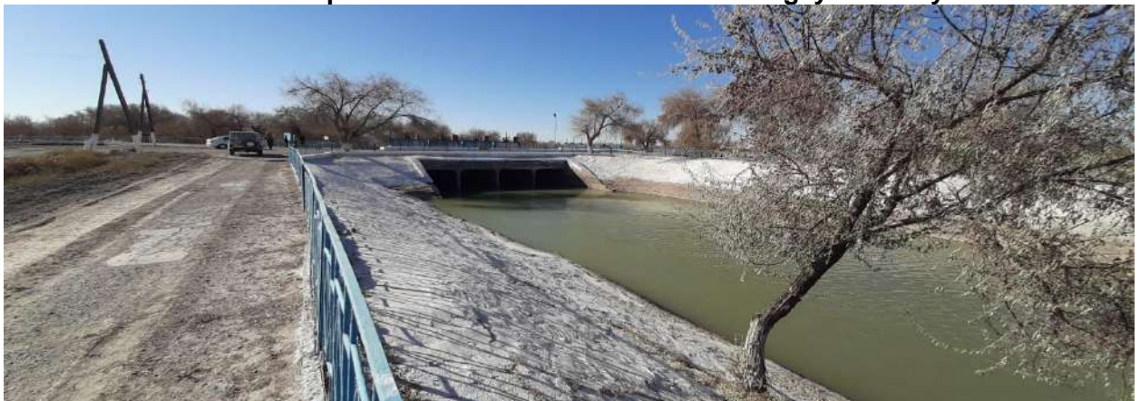
Picture 8D : Downstream pool of the head structure on the Kegeyli Nizhniy Canal
