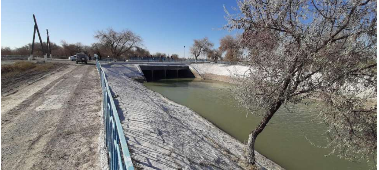
Picture 8B : Downstream pool of the head structure on the Kegeyli Nizhniy Canal
