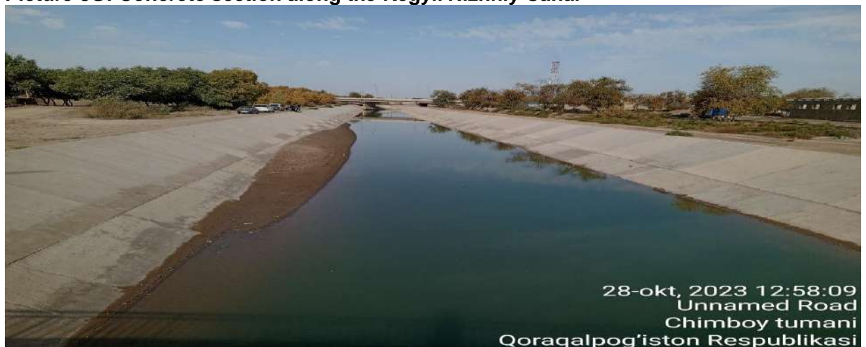
Picture 8G: Concrete section along the Kegyli Nizhniy Canal
