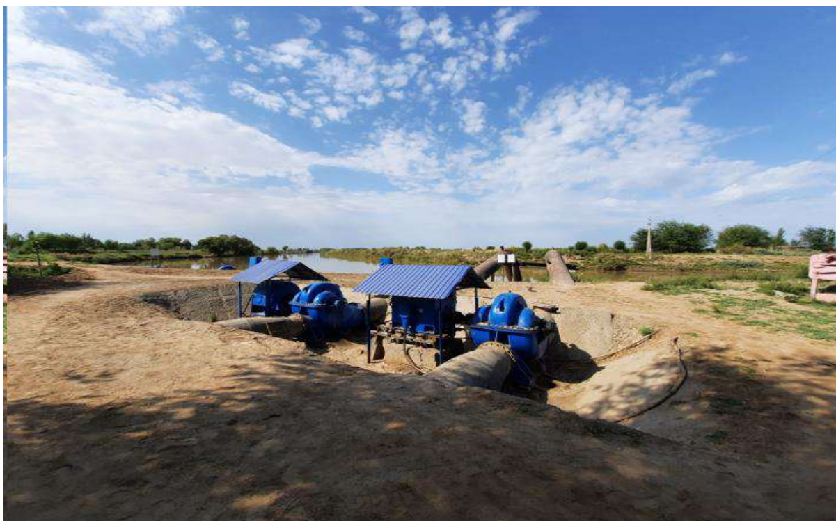
Picture 7: Energy intensive pump used for water withdrawing
