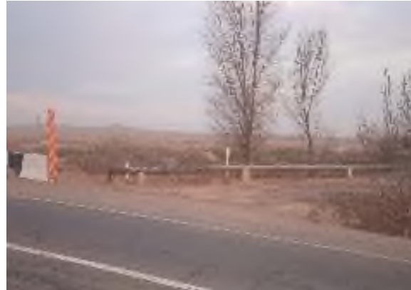
Underground gas pipelines in Termez district (1607km)
