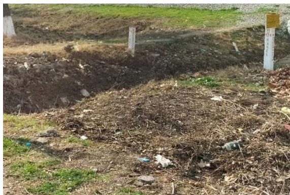
Existing underground cable in Termez district (1618km)
