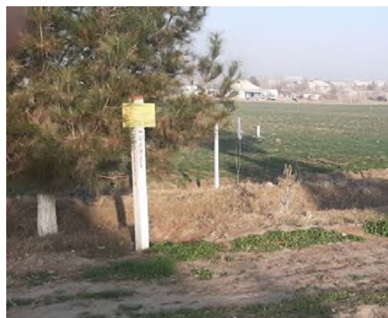
Existing underground cable in Dzharkurgan district (1591-1598km)
