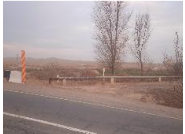
Underground gas pipelines in Termez district (1607km)
