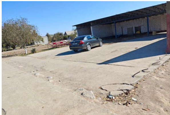
Car wash (only access is impacted)
