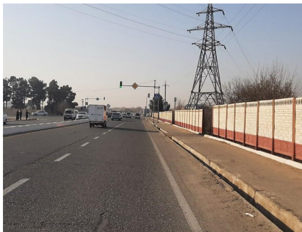
OHTL tower 110 kW in Termez district (will not be affected) – 1616km
