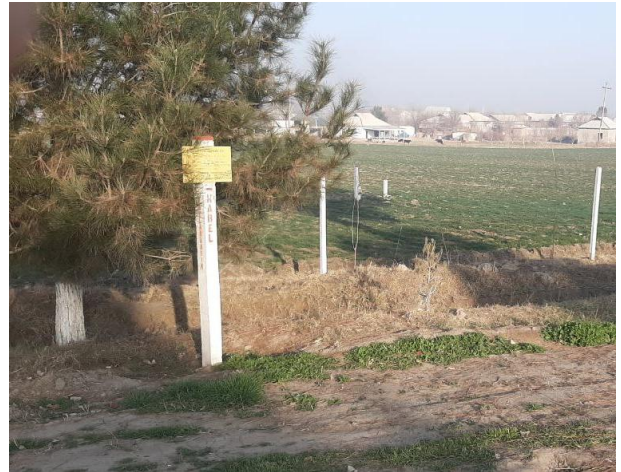
Existing underground cable in Jarkurgan district (1591-1598km)
