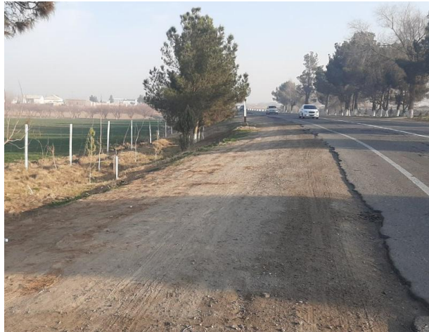
Existing underground cable in Jarkurgan and Termez district (1599-1619km)
