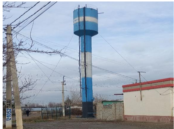
Water tower in Termez district
