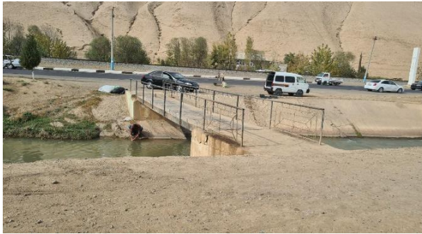
1540 km - The project road runs along irrigation canals and the railway
