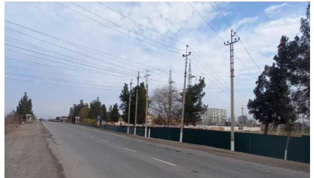
OHTL towers next to the road
