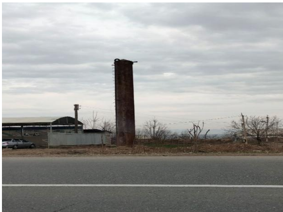
Water tower in Kumkurgan district
