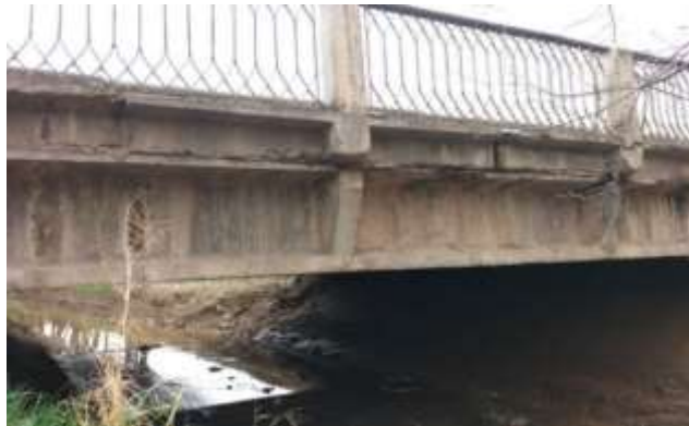
The existing bridge over the Urta Arik canal
