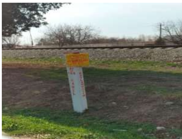
Communication cable in Kumkurgan district (15272km)
