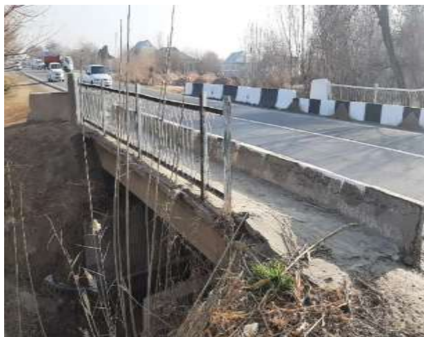
Photo 4: The existing road bridge over Urta arik canal, Termez district
