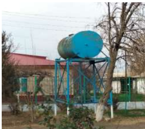
Water tower (on the right side of the road-1525km)
