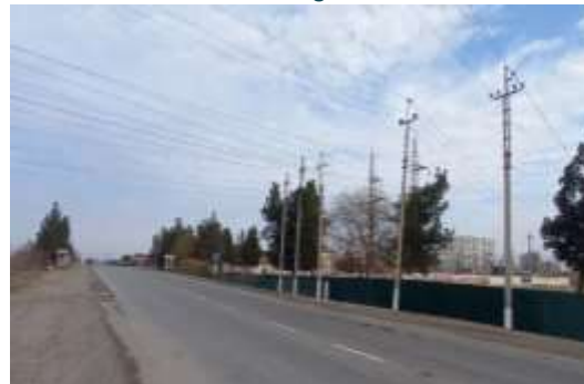
OHTL towers next to the road
