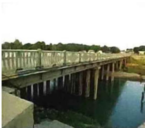
Photo 3: The existing road bridge over Surkhan river, Termez district
