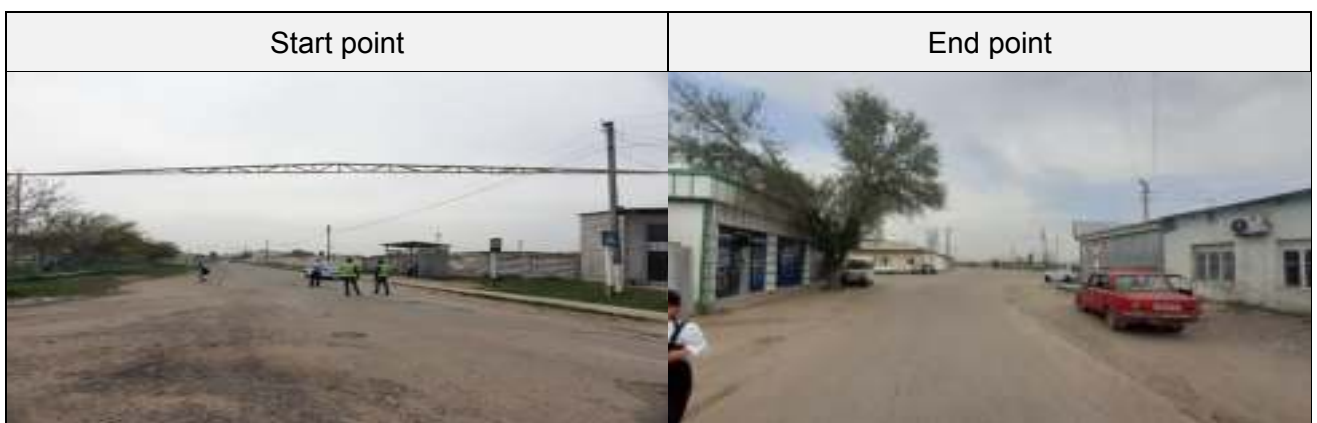
Figure 3. Photos of project road 10V065(4K-768)
