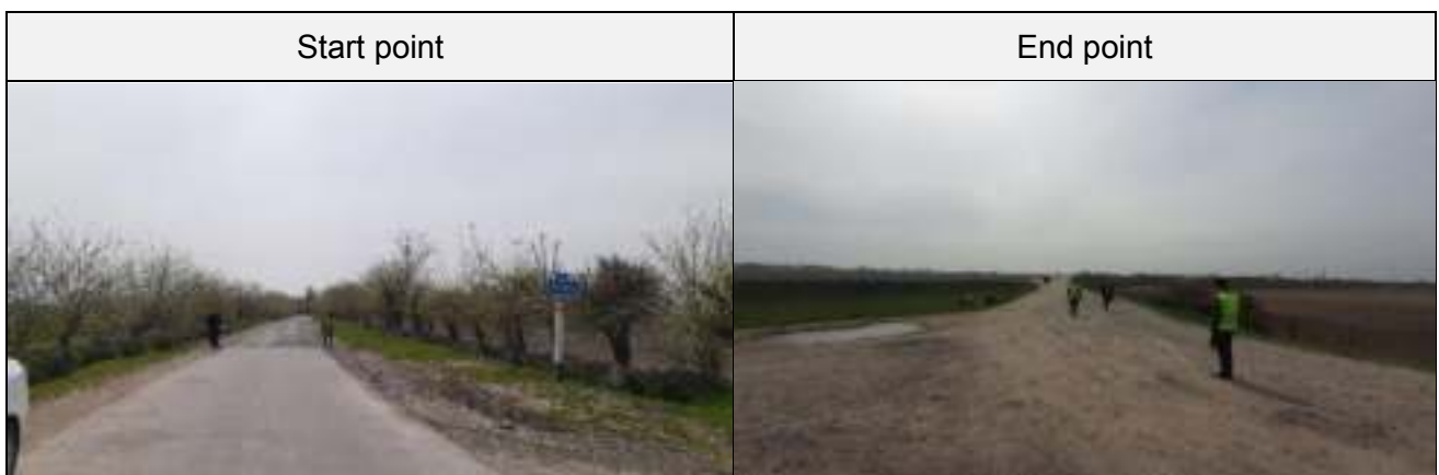
Figure 13. Photos of project road 10V060a(4K-742a)
