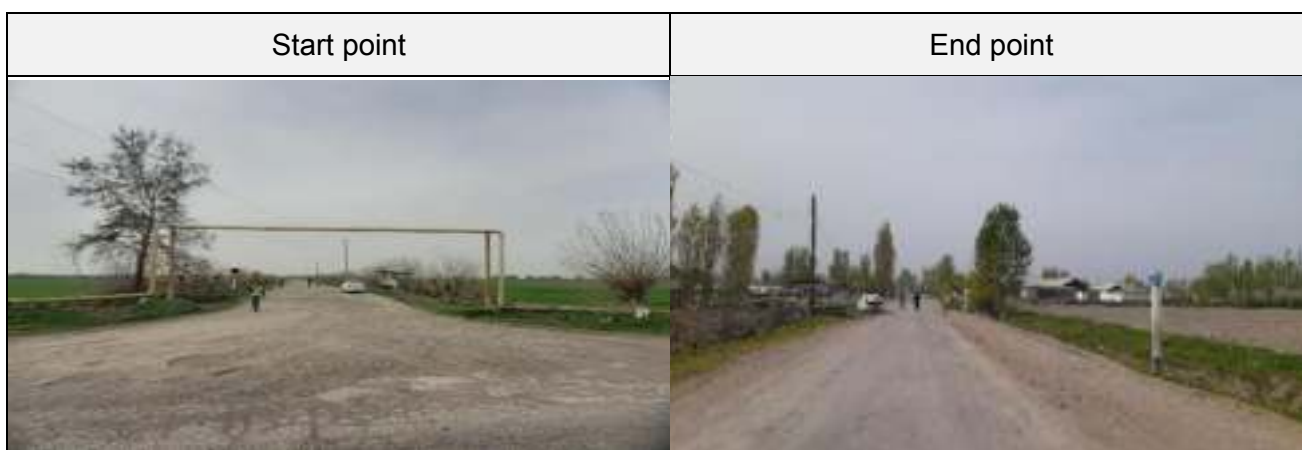
Figure 17. Photos of project road 10V061(4H-716)
