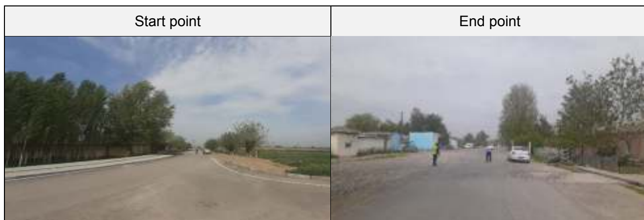
Figure 9. Photos of project road 10V087(4K-783)
