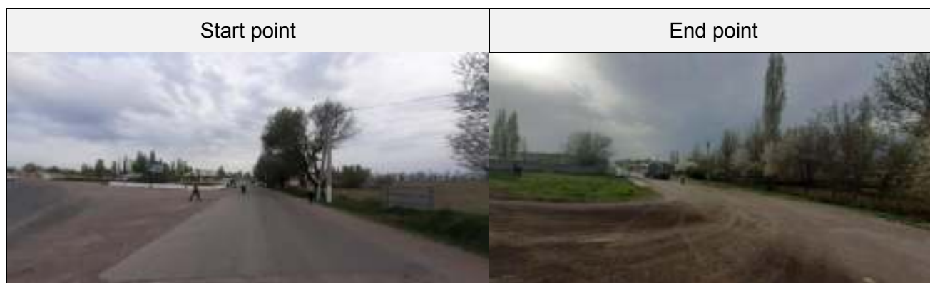
Figure 19. Photos of project road 10V138(4K-721)
