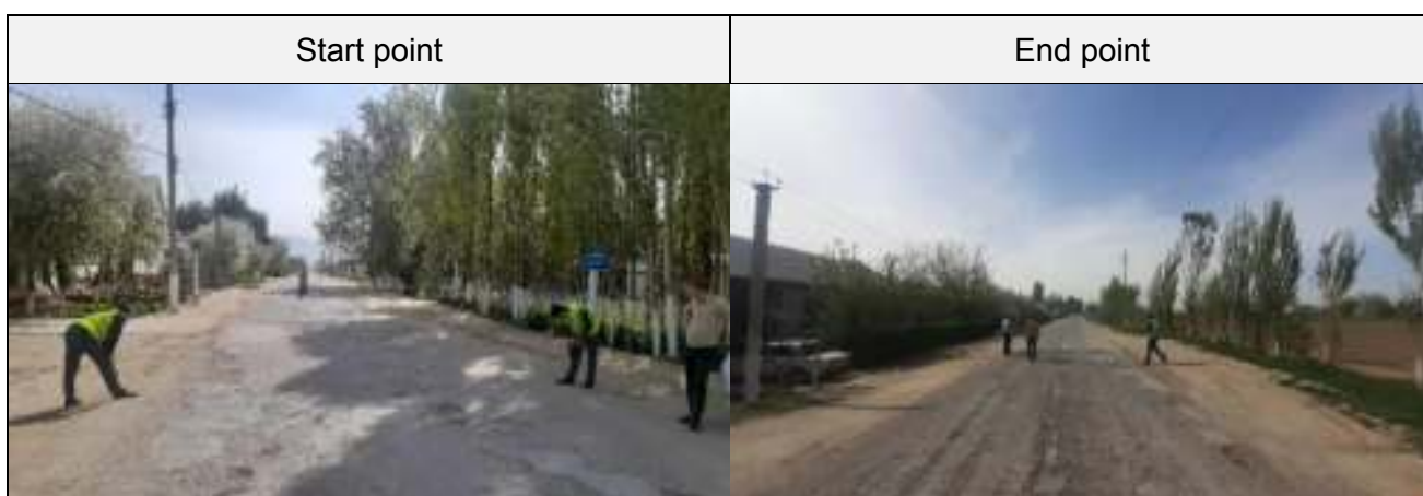
Figure 11. Photos of project road 10V091(4H-731)
